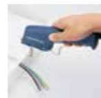
Cutting out small cable channels
