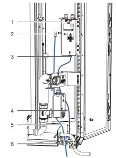
Fig. 61: Connecting the hoses to the LCP
