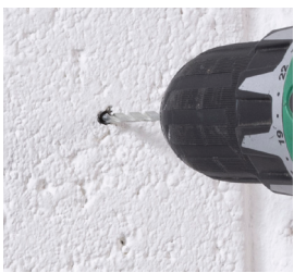
Drill a 5mm pilot hole
