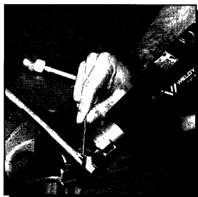
Soldering of copper pipes
