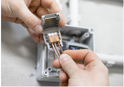
Place the wired connector in the Gelbox.
