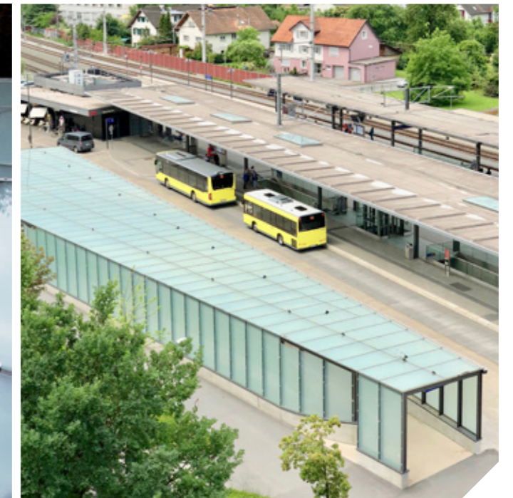
ÖBB train station, Hohenems, Austria – Punkthalter / Point fitting
