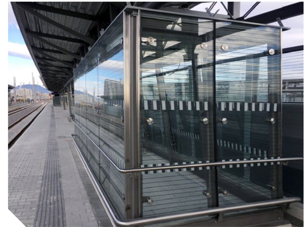
Don Bosco train station, Graz, Austria - Fassadenhalter DISC / Facade fitting DISC
