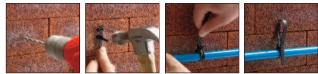
Fixing of Wall Plug Ties.
