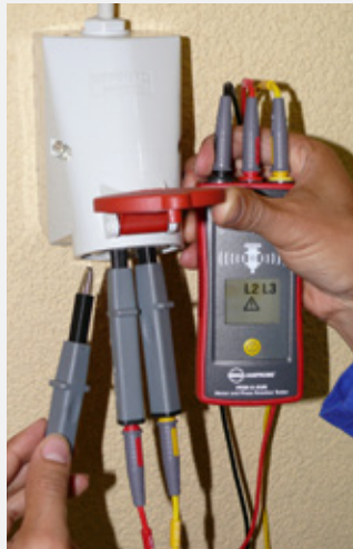
Validate receptacle wiring
