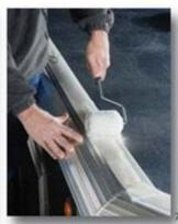
Roll down with a soft roller to conform over contours, seam edges, rivets, or screw heads.
