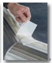
Peel off the protective release liner.
