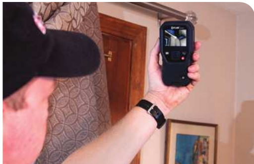
Scanning ceiling & wall joint for moisture issues
