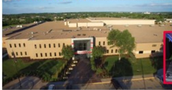
Lincoln, Nebraska Sending Plant
